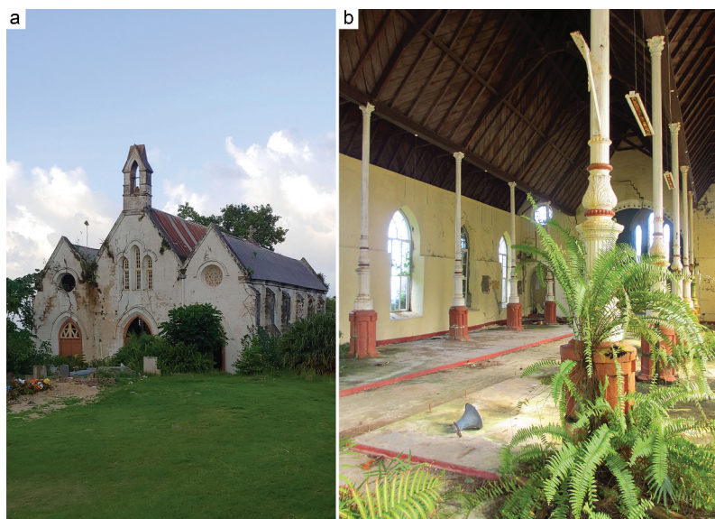
Figure 2. Different views of the St. Joseph's Parish Church: A) View of the crumbling exterior façade from the cemetery and walkway. Photo by Casey D. Allen, 2020. B) Interior of the structure from the southwest entrance. Much of the sunken foundation can be seen on the left of the image. Photo by author in 2020).
